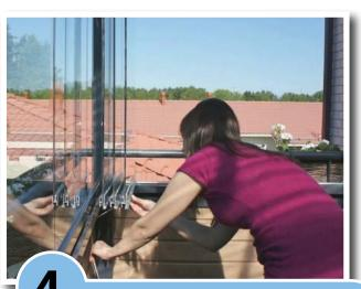
Finish the opening measures by fastening the hook of the wind tie on the sidewall to the groove of the last pane. Tighten the string into the furrow and spin it around the circle part to have the system locked.
